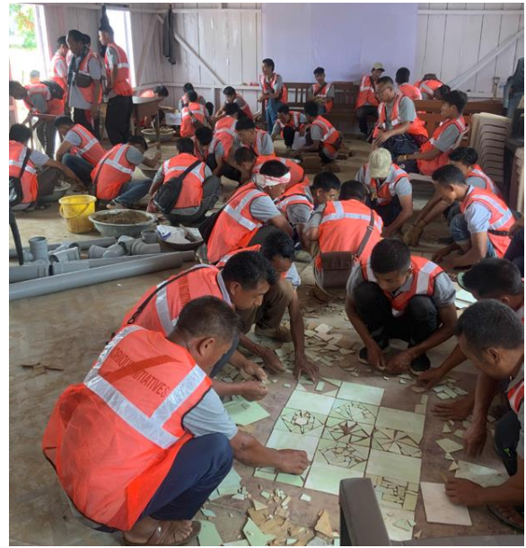
Multi Skilled Technician - Tiling
